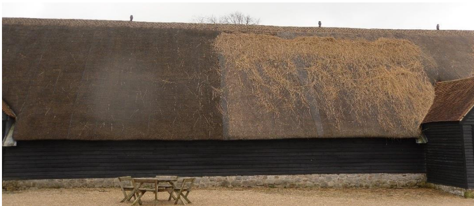
Great Barn. Rear elevation.
